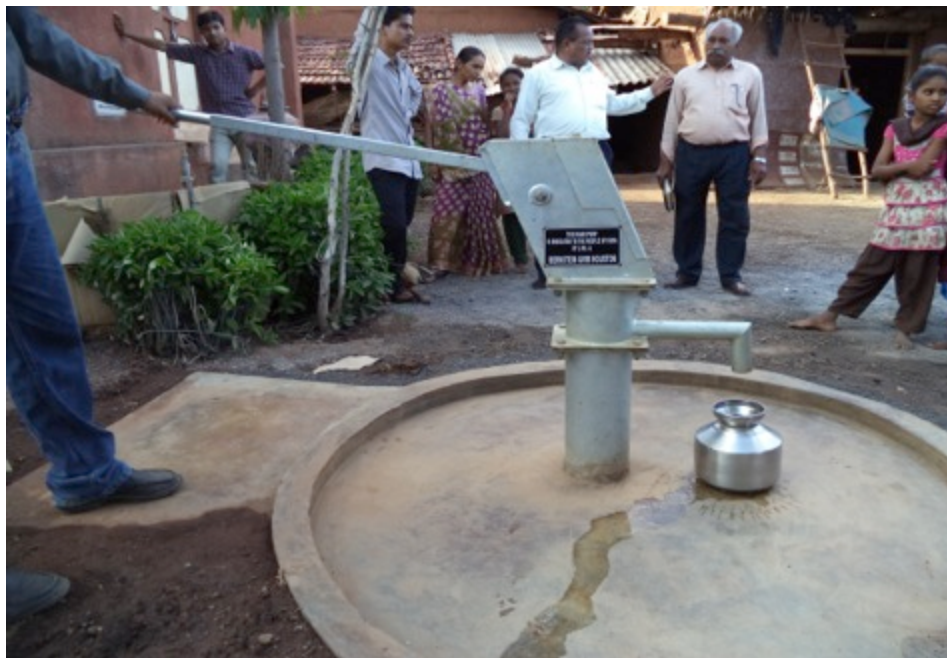
The new India Mark II hand pump is surrounded by a new concrete platform to help keep the borehole protected and mosquitos at a minimum.
