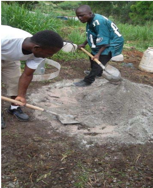
Project in process.
